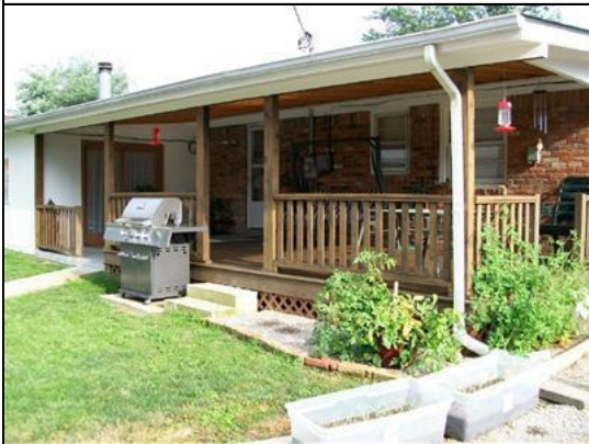
Back View of Covered Deck.
