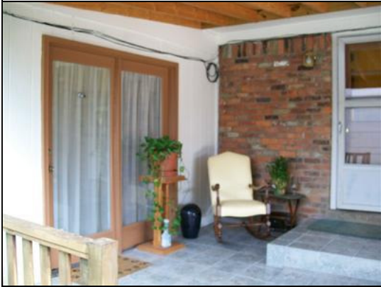
View of Atrium Door from outside.
