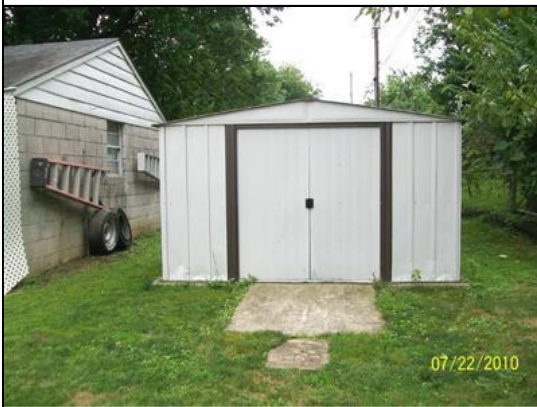
Storage Building is on concrete slab.
